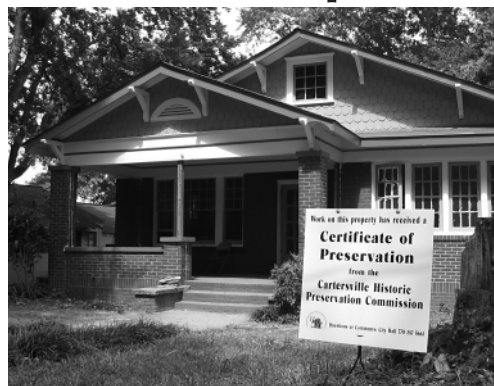
A sign with Certificate of Appropriateness, or in Cartersville, a Certificate of Preservation, notifies the public that repairs or modifications will be taking place on the property.
