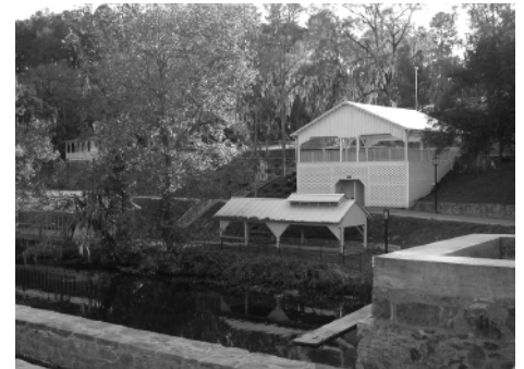
The Augusta Canal Authority is stabilizing the 1845 lock as interpretive ruins and restoring the 1875 lock so that it's operational once again.
